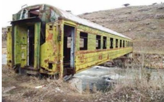
An interesting passenger car, aka bridge.
