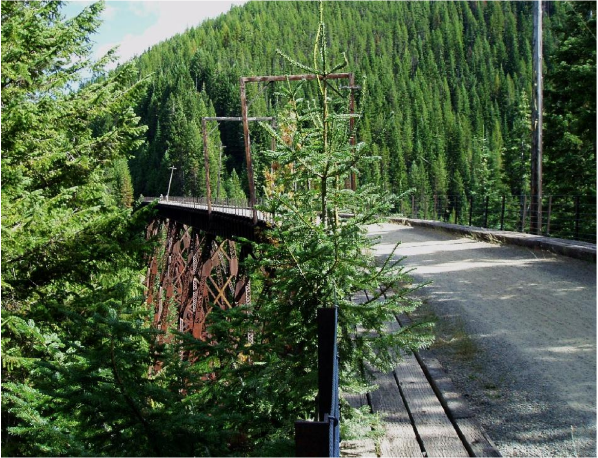
Note the wooden centenary structures still mounted on this trestle
